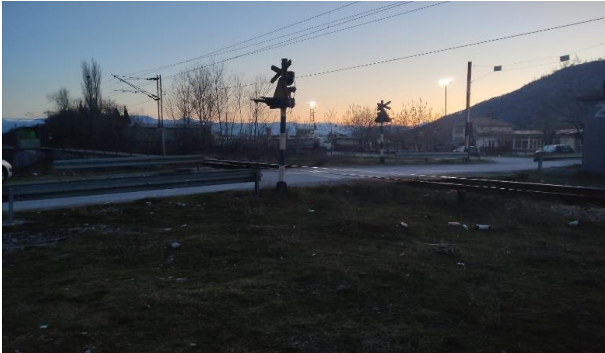
Figure 3: Level Crossing “Morača”
